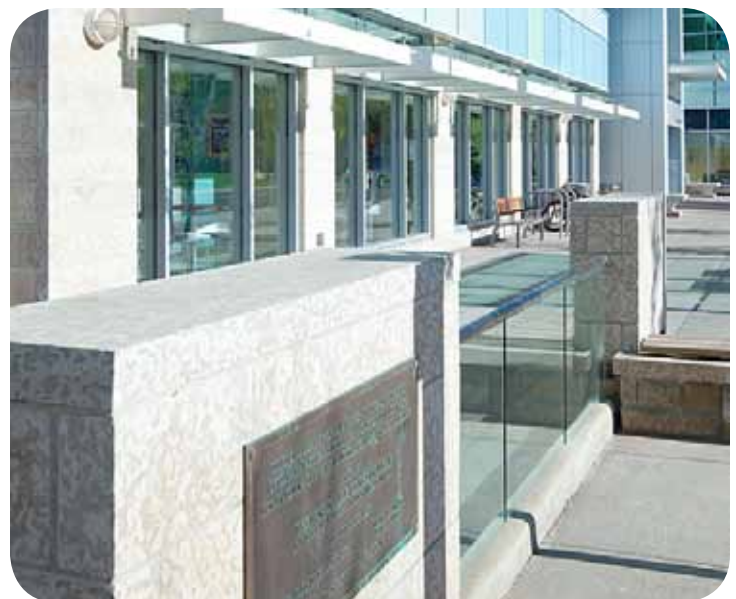
SHELDON CHUMIR CENTRE incorporates sandstone, brick and other architectural elements similar to those used in the veterans hospital that once occupied the site.
